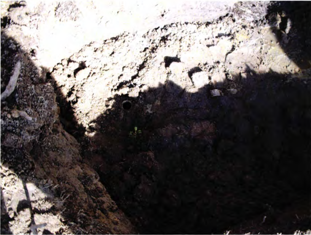
Picture 2: UST 118Banyan in tank excavation.
